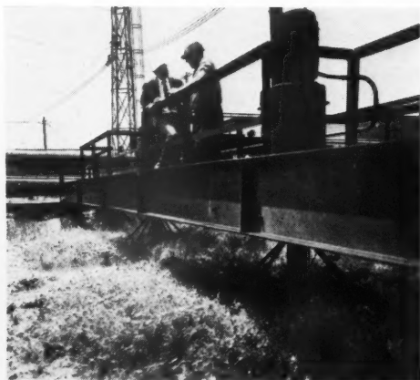
Phenol-eating bacteria need oxygen to live, so we aerate the waste liquids.
